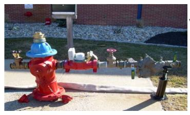
City to hook up to our system and the hydrant will have a meter and backflow prevention device in place to protect our drinking water system from contaminants (below is a typical installation).
